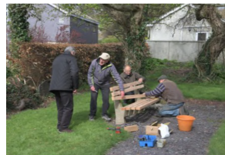
Fitting the new slats, made from Welsh larch, to the concrete bench frames
